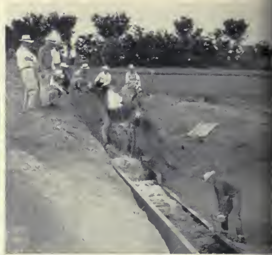
IRRIGATION MADE EASY.—At left, J. A. Fambro, ditch- rider, Carl Duke and Mark Ratliff watch water flowing over lower side of Duke's ditch. Above, Dee Inmon removes a concrete block from his box-type lateral.
